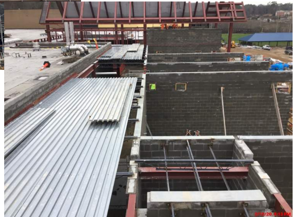
Classrooms – Joists & Decking
